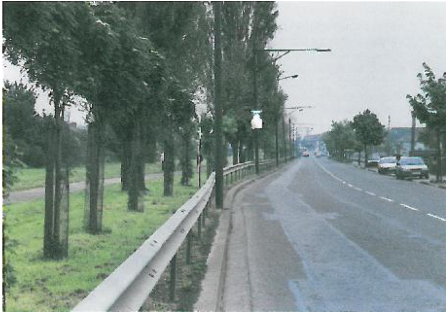
Figure 9.1 Columns placed on the road side of the barrier
