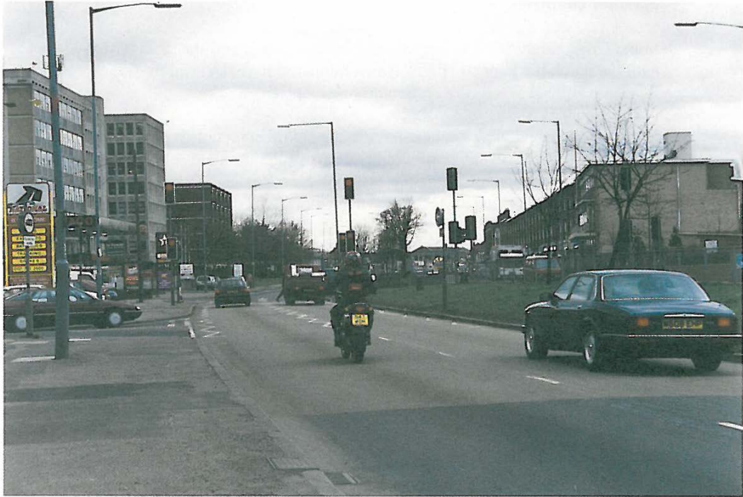
Figure 1.3 Anti-skid surfacing in advance of a junction
