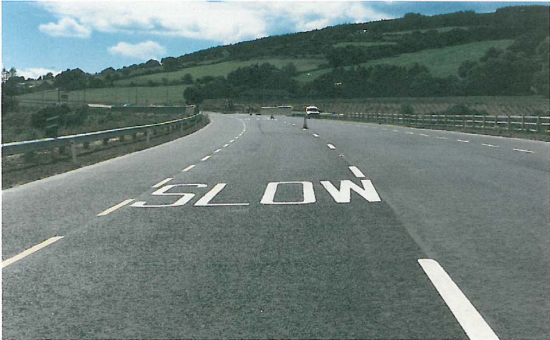
Figure 2.2 Example of a roundabout which is not clearly visible from the approach
