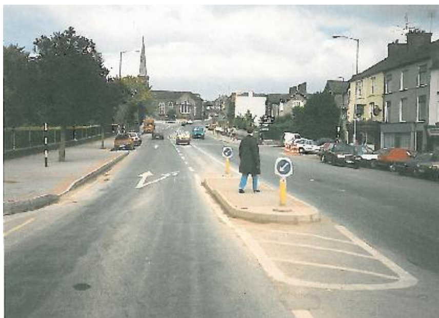
Figure 8.8 Installation of pedestrian refuges and footpath widening in Fermoy
