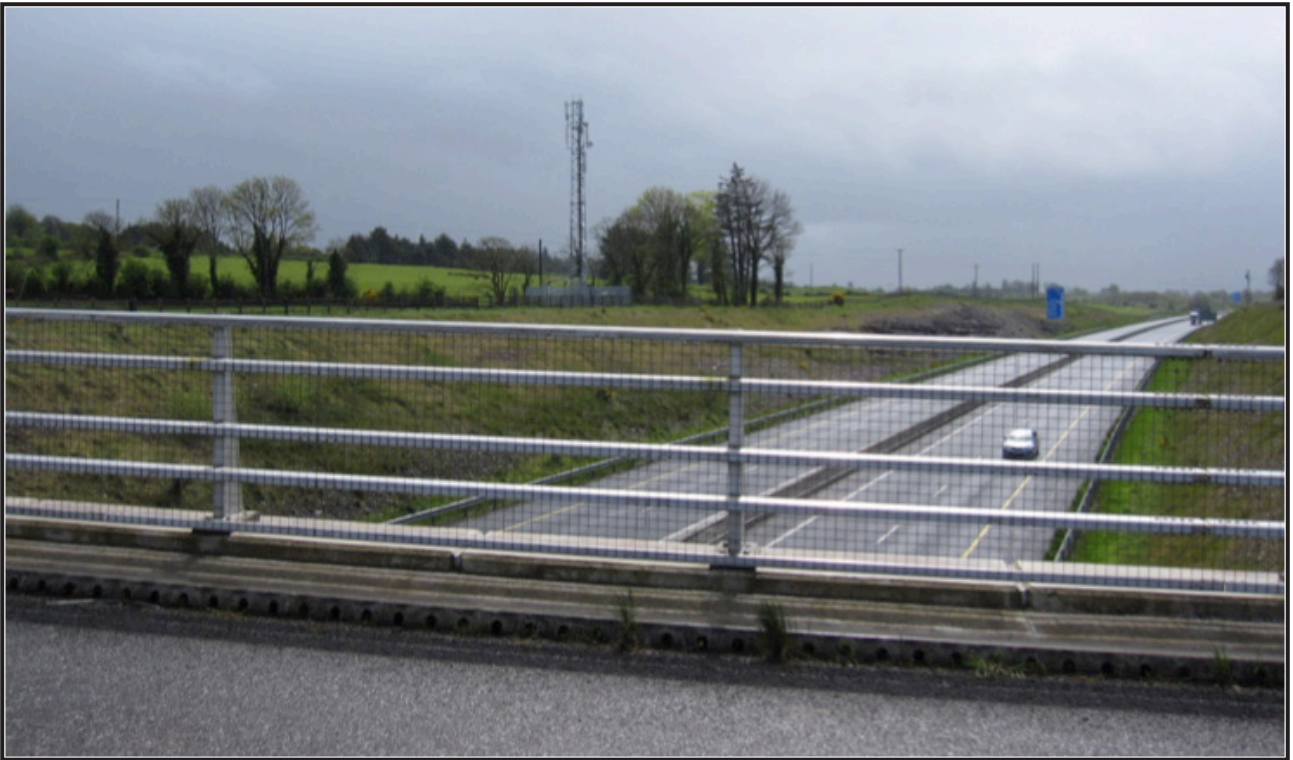
Existing mast from overbridge at Ballynahinch.
