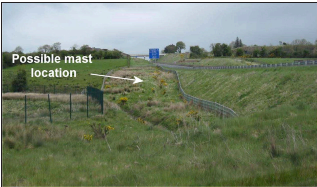
Potential site adjacent to attenuation pond.
