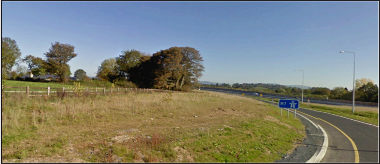
Verge adjacent to eastbound on-slip at Jn 28, Annacotty.
