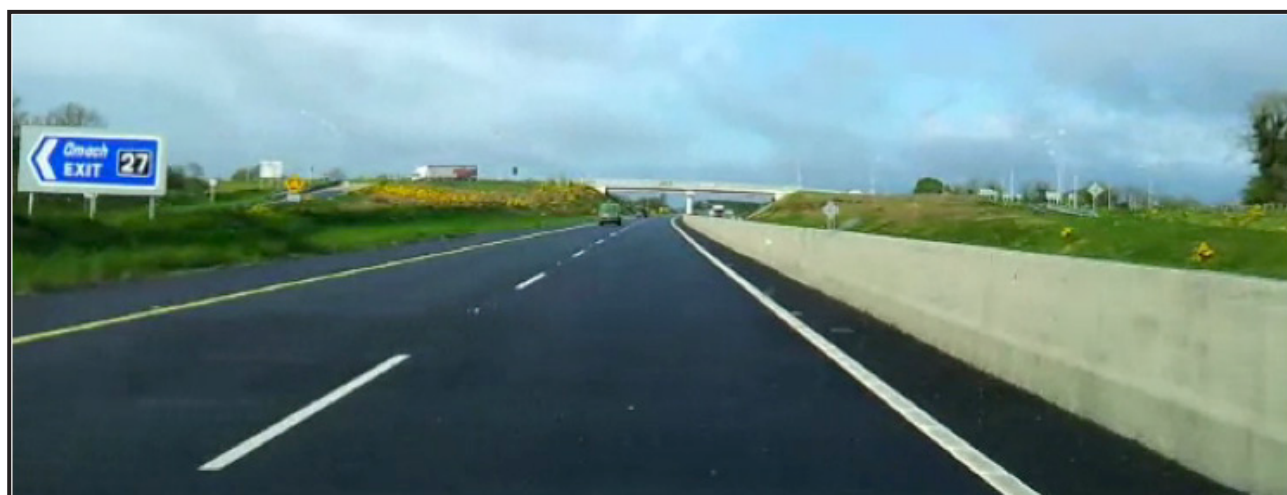
Junction 27, Birdhill from M7 westbound
