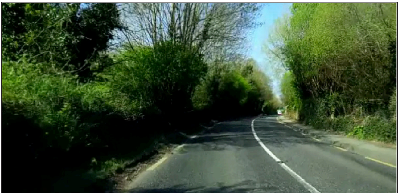
Typical non-improved rural section of N30
