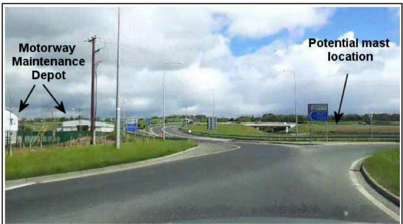
From roundabout adjacent to the motorway maintenance depot;
