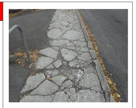
✓ Check – Warrants treatment to strengthen and repair, e.g. removal of surface and loose material, patch and level base and lay new wearing course.
