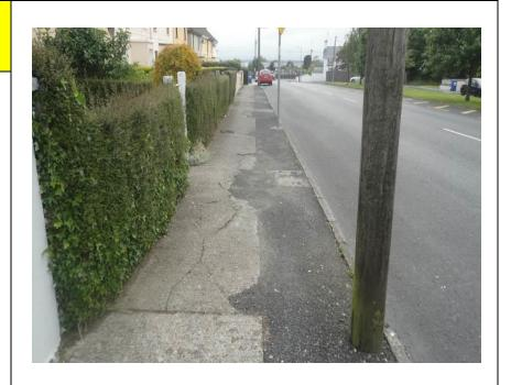
✓ Check – Warrants treatment to prevent expensive repairs being required, e.g. removal of surface and lay wearing course.
