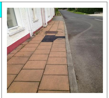
✓ Check – <u>Would only</u> warrant treatment to improve appearance, e.g. replacement of individual paving slabs and relaying of some uneven ones.
