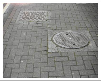
✓ Check – Warrants treatment to prevent expensive repairs being required, e.g. relaying of significant areas of modular pavers.
