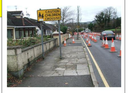
✓ Check – Warrants treatment to prevent expensive repairs being required, e.g. replacement of part of the paving slabs and relaying of others.
