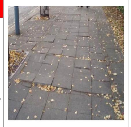
✓ Check – Warrants treatment, e.g. relaying or replacement of the paving slabs across the majority of the rated section.
