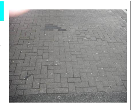
✓ Check – Would <u>only</u> warrant treatment to improve appearance, e.g. replacement of missing or different colour modular pavers.
