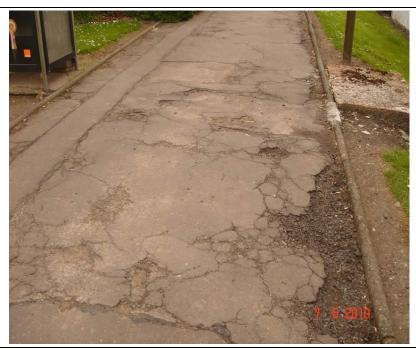
✓ Check – Warrants treatment to strengthen and repair, e.g. removal of surface and loose material, patch and level base and lay new wearing course.
