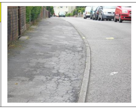
✓ Check – Warrants treatment to prevent expensive repairs being required, e.g. removal of surface and lay bituminous wearing course.
