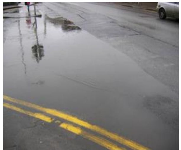
Significant ponding at a busy intersection creating potential safety hazard.
