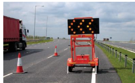
Figure 3.9: Mobile VMS (Displaying Chevrons)
