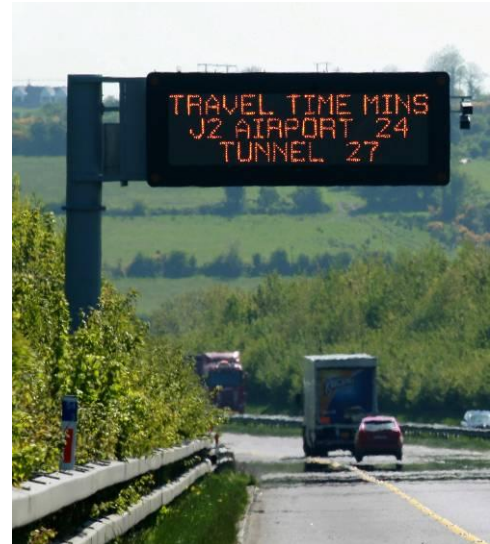
Figure 3.3: Typical LED VMS (Continuous Matrix)
