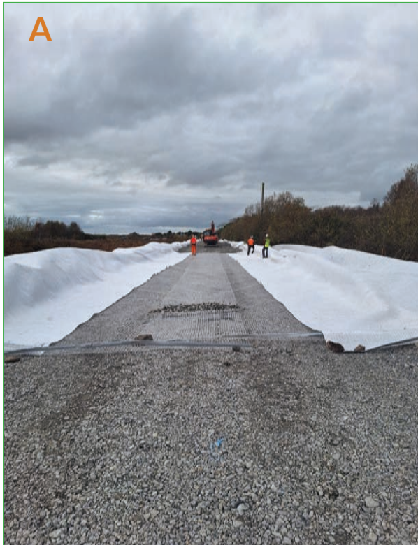
Figure 4.9 - Installation of transverse woven white geogrid (A), and longitudinal biaxial polypropylene type geogrid (B) on the R400 in Co. Offaly in October 2024
