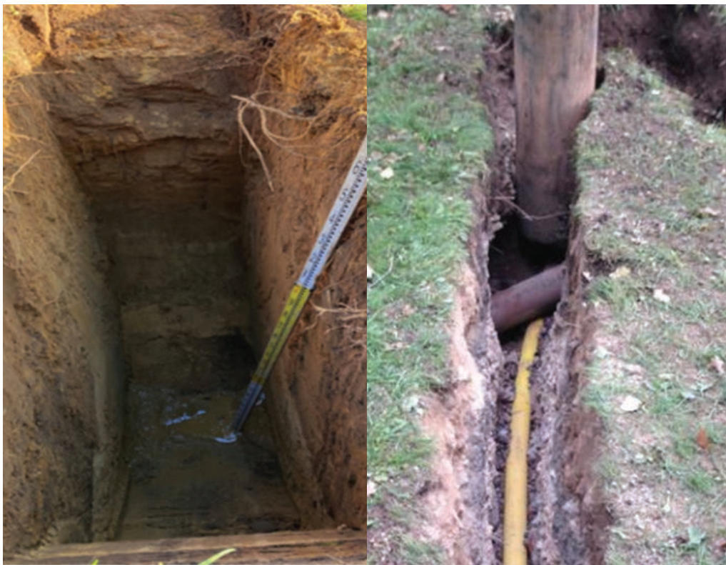
Figure E.1.2 – Trial Pit (left) and Slit Trench (right)
