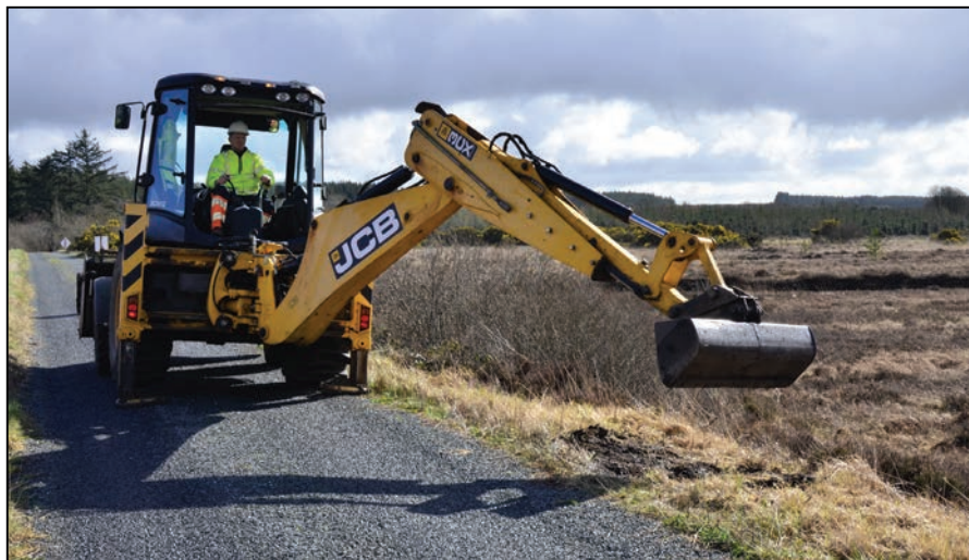
Figure 3.5 - Showing maintenance, opening of water cuts
